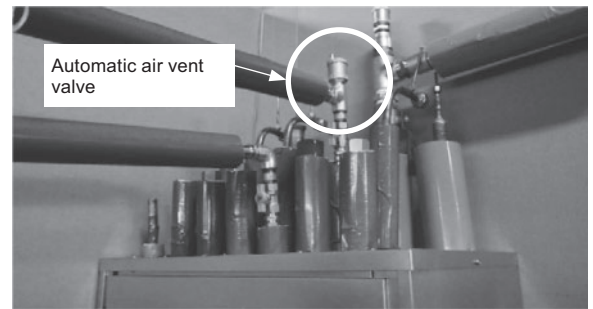
Figure 1 Automatic air vent valve
